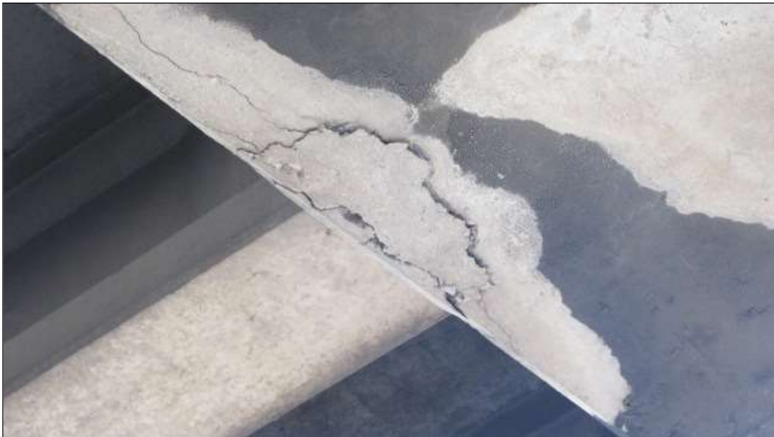
SPALL FORMING BTWN. COLUMNS 2 AND 3 AT BENT 1-2' W X 18" LONG.
