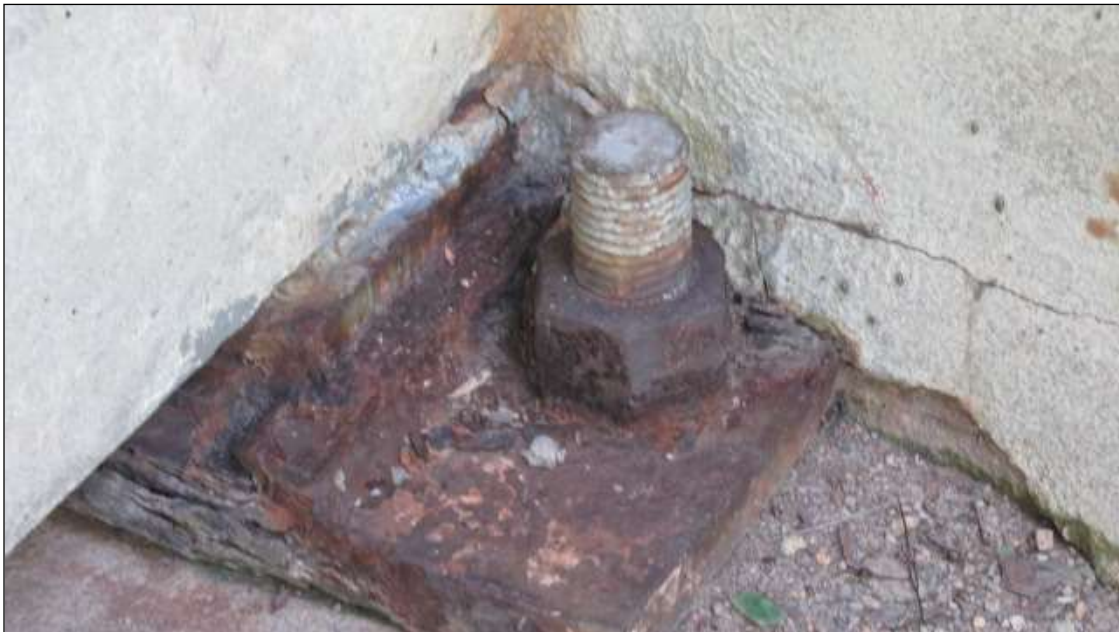
THE EXTERIOR BRGS AT THE ABUTS. SHOW SURFACE RUST WITH 1/16" DEEP PITTING.
