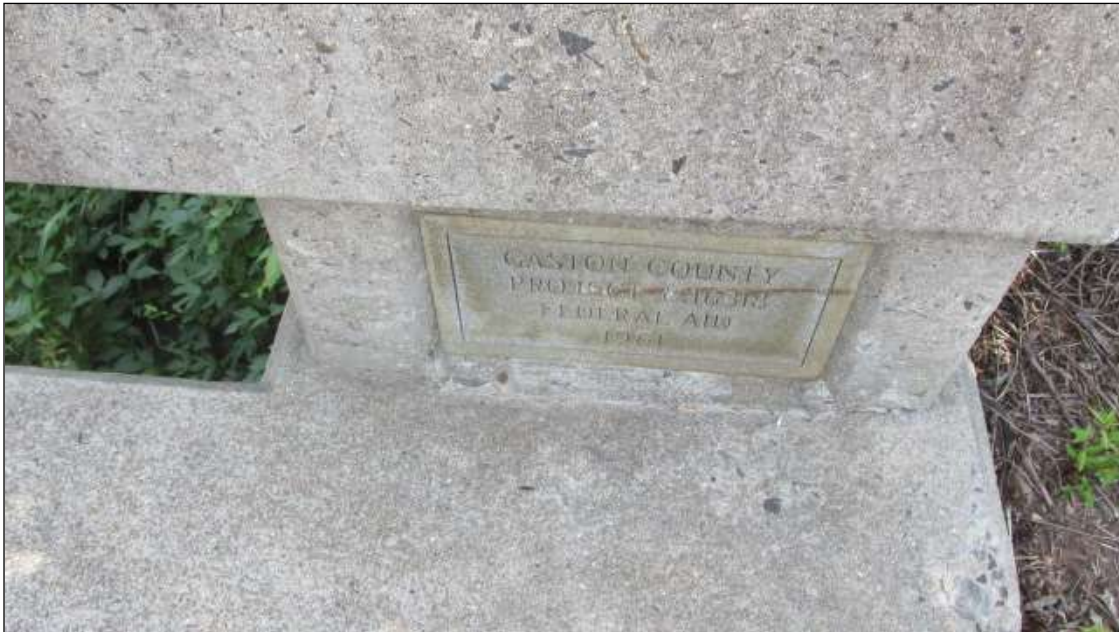
INFOR. PLATE AT THE NORTHEAST CORNER
