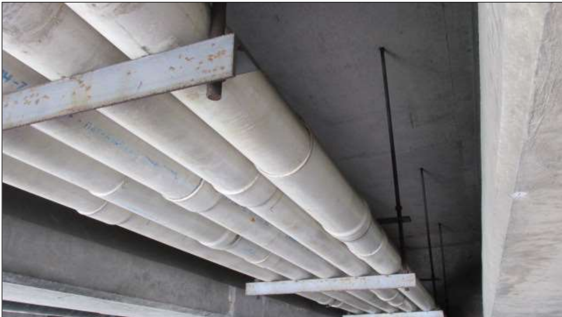
UTILITY IN BAY 8
