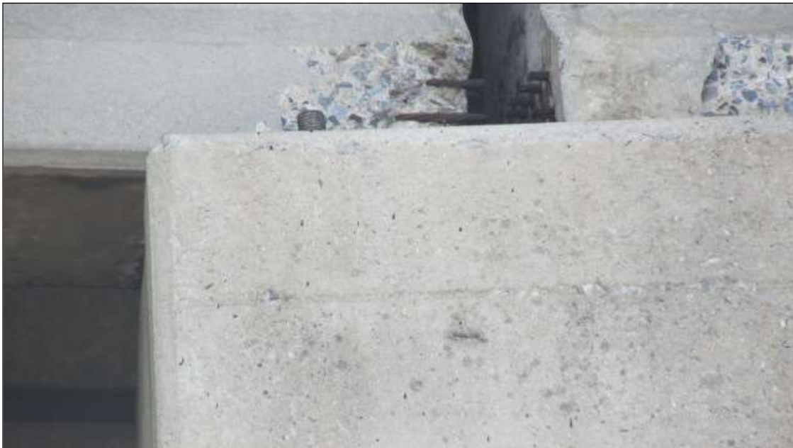
SPALL ON THE EXTERIOR GIRDERS AT THE INT. BENTS WITH STEEL EXPOSED FOR 3" L X 2" HIGH.
