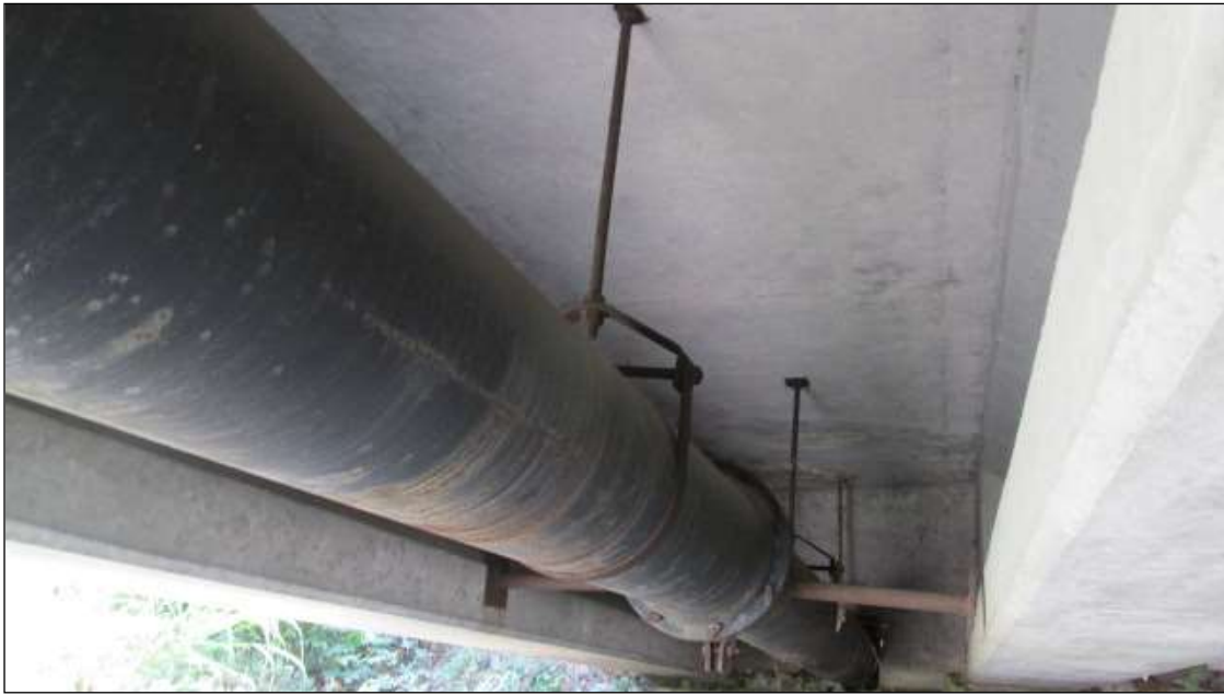
UTILITY IN BAY 7
