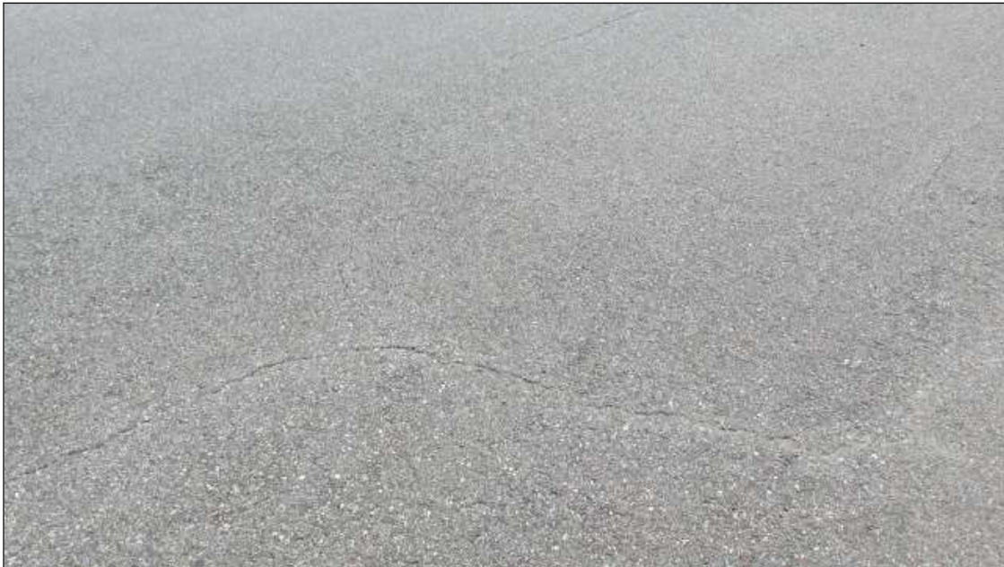
TRANS. CRACKING CRACKING IN THE ASPHALT WEARING SURFACE IN SPAN 1. SIMILAR IN SPAN 2 AND 3.
