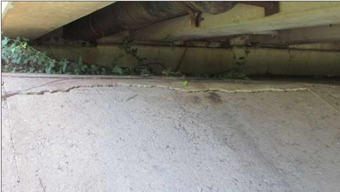
CONCRETE SLOPE PROT. CRACKED AT THE TOP FOR 15' HORIZONTALLY.
