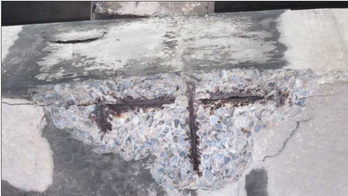
SPALL 3' L X 2' WIDE X 1" DEEP WITH REBAR EXPOSED ALONG THE BOTTOM OF BENT 1 CAP IN BTWN. BAYS 1 AND 3.
