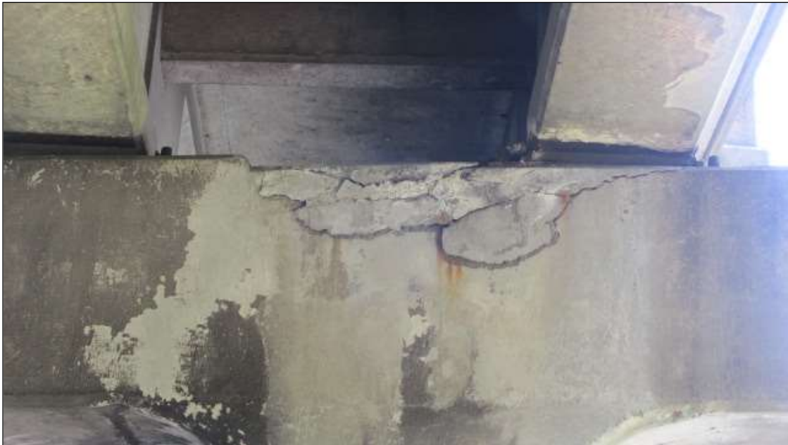
SPALL FORMING ALONG THE TOP CORNER OF BENT 1 CAP WEST FACE 10" HIGH X 32" WIDE, BTWN. BEAM. 8 AND 9.
