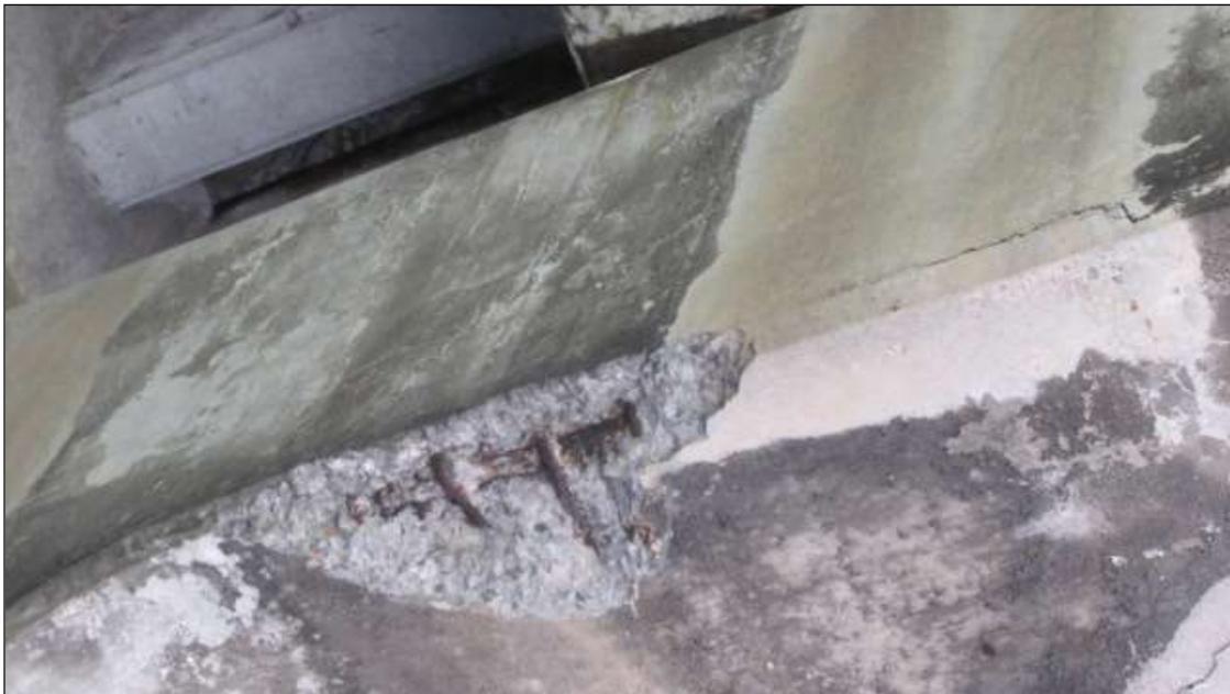
3' WIDE X 1' LONG SPALL BTWN. COLUMNS 1 AND 2 WITH REBAR EXPOSED AT BENT 3.
